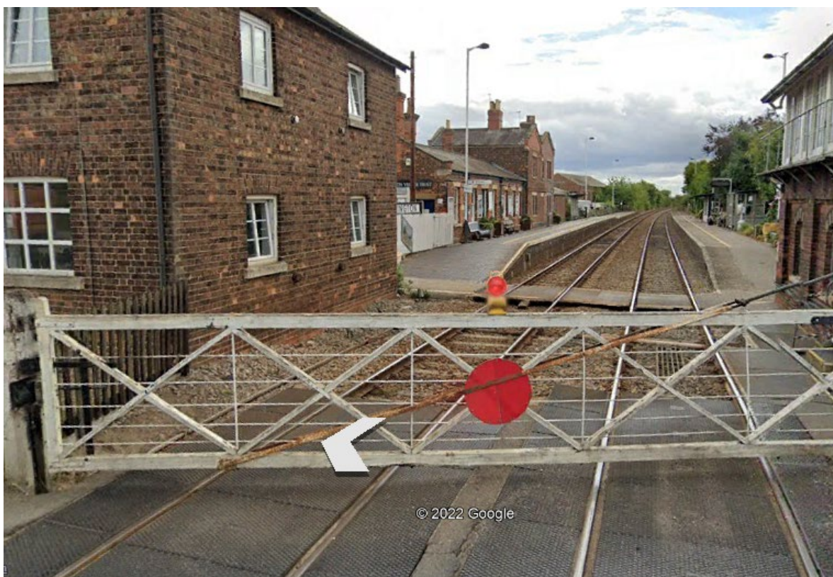
Figure 17.6 - Heckington Station Line Crossing Facing East to Illustrate Screening from Rail 2 to Energy Park 7
