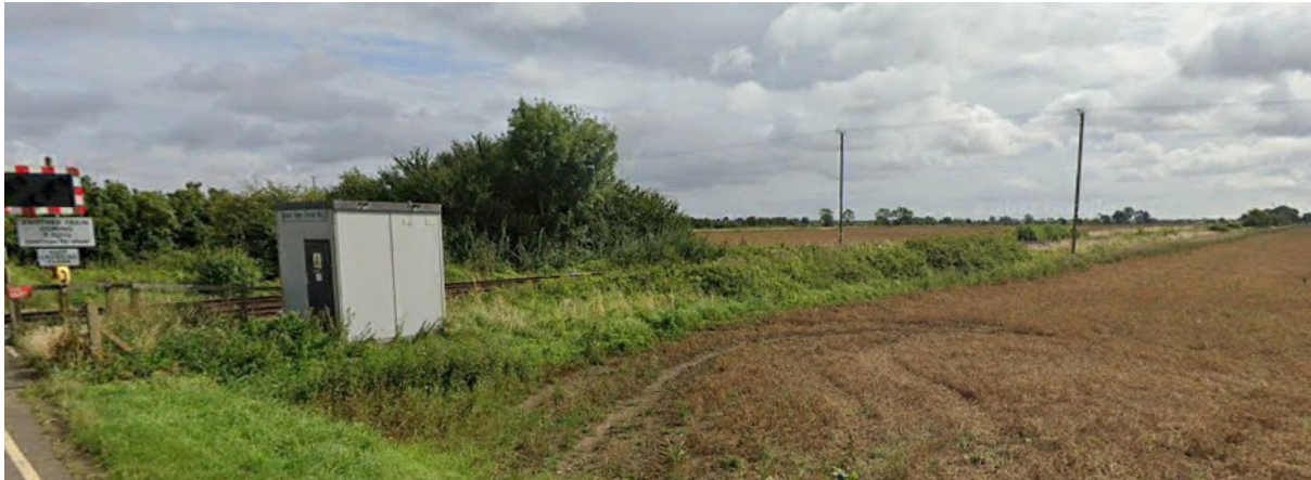
Figure 17.7 - Great Hale Drove line crossing (orientation northeast) illustrating the screening present for Rail 2 and Energy Park 8
